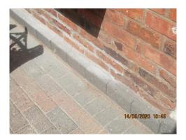
Brickwork to all elevations is generally pointed in a in a sand and cement mortar although there is some localised evidence of lime mortar. The original pointing in a property of this age is likely to have been lime mortar. Sand cement mortar is inappropriate and may be causing damage to the timber frame.
