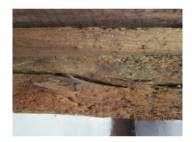
Evidence of timber infestation was noted around the property to timber beams and roof timbers.
