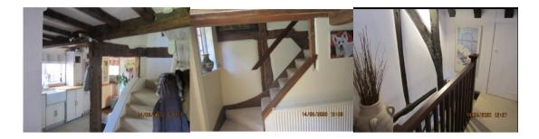
Whilst the staircases were found to be twisted and uneven they were generally firm underfoot and considered to be in functional order. There is no outer handrail to the lower section of the staircases leading from the utility room and kitchen, this does not comply with current regulations and is considered to be hazardous.
