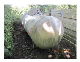
The property is served by and LPG system with gas storage tank located within the garden. We have seen no service history for the LPG tank and recommend that it is serviced in accordance with installers guidelines.
