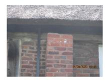
To the left side of the property there is a brick built chimney stack however this has been reduced below the eaves level and capped. The chimney flu is now redundant. The redundant flu should be ventilated at the top and bottom to guard against condensation occurring within the sealed flu.
