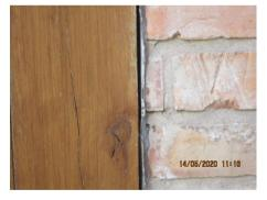
The seal at the base of the door frame is missing and should be finished. Evidence of dampness was noted at the base of the outer wall however this appeared dry at the time of inspection was considered to be historic in nature. Window frames to the left and right side elevations protrude beyond the line of the face of the brickwork and are not fully sealed.
