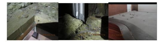
Evidence of vermin infestation in the form of droppings and damage to insulation was noted within the roof void and within some habitable rooms. Pest control specialists should be asked to advise on method or eradication.
