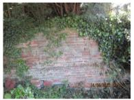
The party boundary wall to the right of the site is formed from solid brickwork. The wall is in poor condition, shows severe weathering and structural damage due to the proximity of trees. The wall requires extensive maintenance and the trees will need to be removed to prevent further damage.
