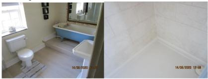
The fittings and appliances in the left side guest bathroom are of mixed age but were found to be in serviceable order. There is evidence of the use of flexi-trim to the seal around the shower cubicle. There may be some hidden defects to the timbers below. Defective seals should be made good and you should anticipate that some repair may be necessary to these areas when fittings are removed.
