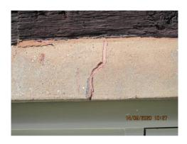
There is a concrete lintel spanning the ground floor window frame to the right side of the property. The lintel has cracked and has been filled with mastic sealant. The lintel requires replacement.
