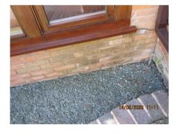
There is evidence of damp staining at the base of the outer walls which appeared to be dry at the time of inspection and may be the legacy of historic problems. Rainwater goods should be subject to routine maintenance to include clearing debris resealing joints and realignment as necessary.
