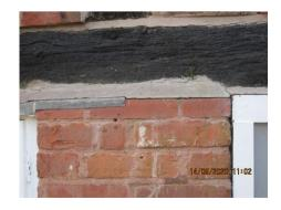
Window/door frames are not fully sealed which will mean they are not fully watertight and may be prone to water penetration. (the use of silicon based sealant is likely to be prohibited). The lead flashing above the Utility window frame may trap moisture against the timber and cause rot. The lead flashing should be removed, window frame re-sealed and defective joinery repaired as necessary.
