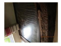
There is evidence of the original wattle and daub in a display panel located in the central stairwell. The extent of wattle and daub to walls and ceilings cannot be confirmed and its maintenance will be a requirement of the listed status. It should be noted that original wattle and daub contains organic matter which will be considered to be a biological hazard and a possible source of anthrax. You are advised to seek professional advice on this matter.
