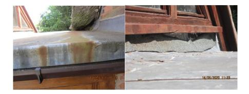
There is a flat lead roof covering to the section between the original building and the extension. The roof covering shows light rusting but no signs of water penetration was noted to the ceiling below. The roof covering is considered to be in serviceable order. There is a mineral felt flashing between the flat roof covering and the extension. A section of the flashing has dropped and requires re-fixing.
