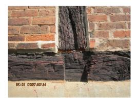
Evidence of the use of expanded foam filler was noted around some joints however this is not considered to be consistent with the listed status of the building.
