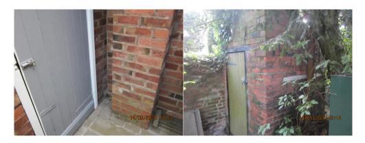
The brick built boiler store shows general wear and tear but was considered to be in serviceable order. The roof covering requires overhaul to include, repairing defective tiles and fitting rainwater goods. Defective joinery requires repair.
