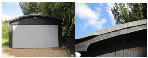
There is a detached double garage being of timber frame construction with curved felted roof and timber up and over door. The timber frame shows general deterioration and requires routine maintenance. The felt roof is loose fixed and requires refixing/overhaul. Eaves gutters are congested and require overhaul.
