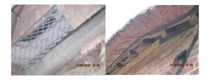
Timber soffit boards within the eaves are fitted with ventilation openings. The ventilation openings vary in size and are covered by a variety of metal mesh which varies in gauge. The larger gauged mesh may allow access by birds, bats or other vermin.
