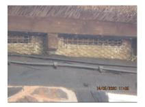
It was noted that the soffit boards to the rear elevation, above the door, are formed from a material that may contain asbestos. Comments made later in this report relating to asbestos containing materials should be noted.
