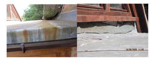
The flat lead roof covering shows general weathering but no signs of water penetration was noted to the ceilings below and was considered to be in serviceable order. The felt flashing to the gable has slipped and requires re-fixing. All flat roof coverings have a limited lifespan and will require repair/maintenance from time to time.
