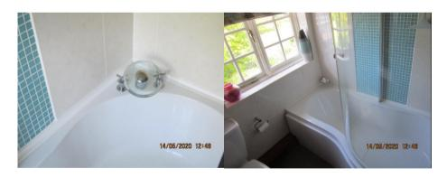
The fittings and appliances in the central guest bathroom of of mixed age but were found to be in serviceable order. There is evidence of the use of flexi-trim to the seal around the shower/bath cubicle. There may be some hidden defects to the timbers below. Defective seals should be made good and you should anticipate that some repair may be necessary to these areas when fittings are removed.
