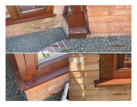
Timber window frames were regarded as being generally well decorated however there is some evidence of general weathering along with deterioration of joinery and past repair. Frames are not flush to adjacent brick walls and are not fully sealed. Mastic seals have split and require re-sealing.
