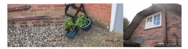
There is some evidence of damp staining at the base of the outer wall to the rear elevation and above the flat roof which suggests that the clearance is not adequate. The amount of clearance provided should be discussed with the thatched when the roof is next replaced.
