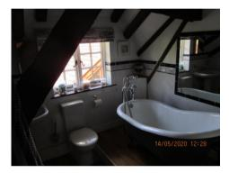
The fittings and appliances in the main en-suite bathroom are of modern design, show some wear and tear but were found to be in serviceable order. The column bath tap requires reanchoring and cold tap requires easing. The bathroom would benefit from and extractor unit.
