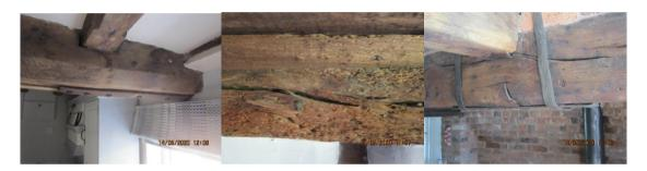
A feature of the property are the original timber beams and joists, these show signs of distortion, past cut and repair, strengthening as well as evidence of timber infestation. These beams are an important feature of the property and would form part of the listed status. Given the nature and age of construction the beams appeared to be performing adequately at the time of inspection.
