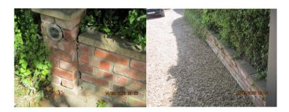
The garden walls adjacent to the rear drive to hardstand shows sign of impact damage and requires repair. Garden walls within the site are generally built from single leaf brickwork. We are unable to confirm that the retaining walls around the site are constructed to an appropriate specification although they appear to be adequately fulfilling their function at the time of our inspection.
