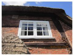
The timber lintel spanning the window frame first floor to the right side elevation is under sized and requires upgrading.
