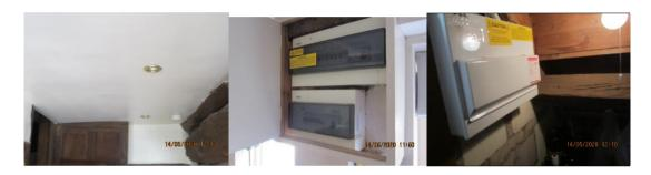
Some adaptations appear to have been made that will have required certification by an Electrician (e.g., replacement consumer units, spot lighting, extension wiring). The systems appear to be past their periodic inspection date (circa May 2018) The Institute of Electronics and Technology (IET) recommends that electrical systems are inspected and tested every ten years and upon every change of occupancy. You should ask an appropriately qualified person to inspect the electrical system now.
