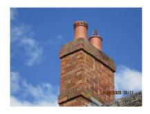
The left side chimney stack is constructed from brickwork with stepped lead flashing and two clay pots. The chimney stack shows signs of general weathering but was considered to be in serviceable order. One chimney pot is fitted with an open grill cage and one with a clay terminal.
