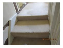
The short rise to the top step to the reception room staircase is a trip hazard and does not conform to current regulations.
